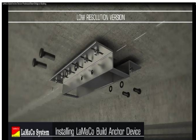
9] Install & Fix the Side Bolt & Nut
