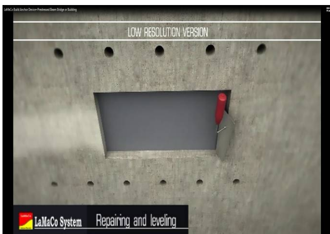
5] Patching to Leveling
