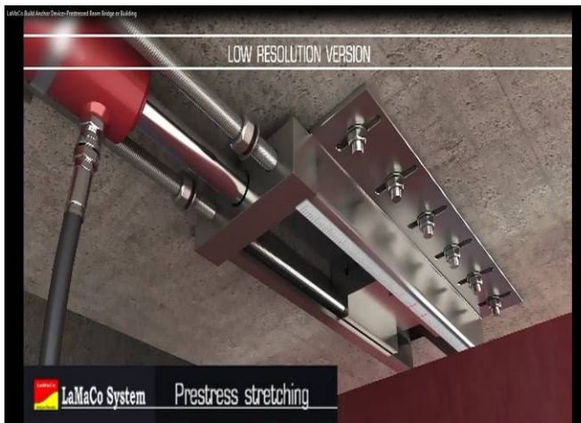
15] Jack Pump for Prestress Stretching
