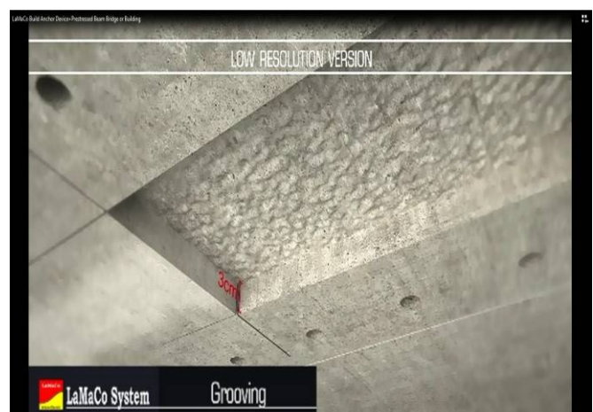
4] Hack Out or Grooving, Depth Set 30mm
