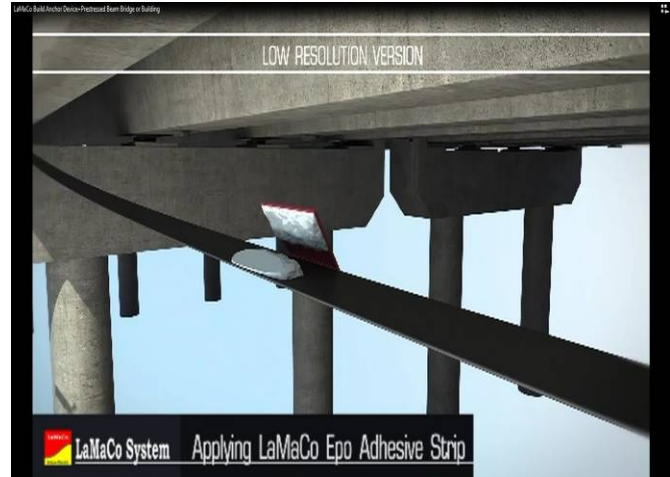
14] Laying the LAMACO-Epo Adhesive Strip
