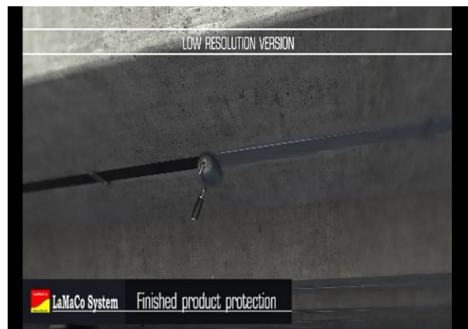
18] Fireproofing Protection on Build Strip PB
